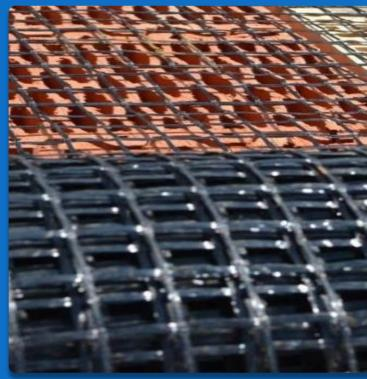
Reinforcement of horizontal seams of masonry walls erected in seismically hazardous regions in order to increase the bearing capacity of masonry.
